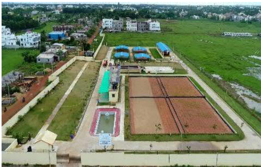
Septage Treatment Plant
