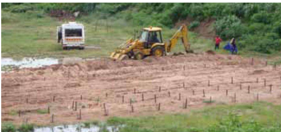
Figure 4-9: -Typical deep row entrenchment site
