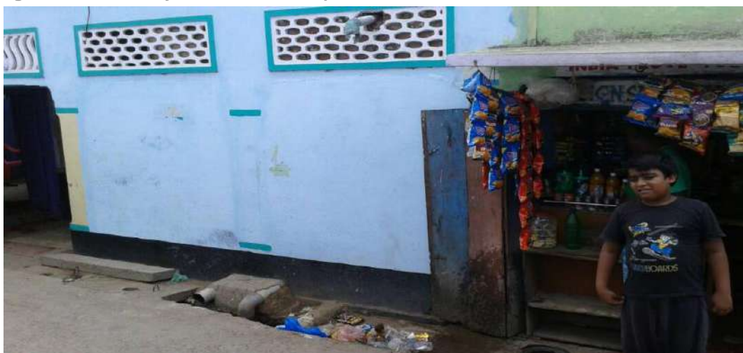
Figure 2-3: -Insanitary household toilet open drains
