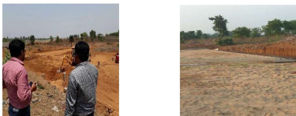
Figure 4-11: SeTP site being excavated for foundation
