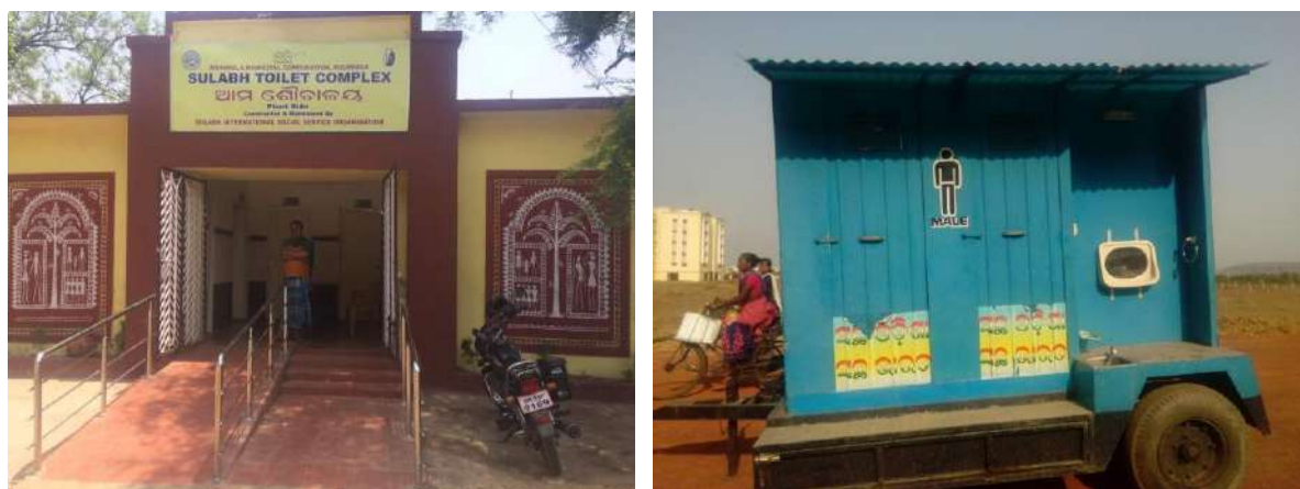
Figure 4-5: -Hybrid toilet at Rourkela Steel Plant Site and mobile toilet at BPUT construction site
