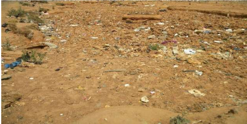
Figure 4-12: Temporary Disposal of sludge were the sludge has been covered by soil
